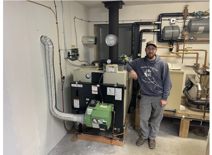
Facility Manager Collier Hard
